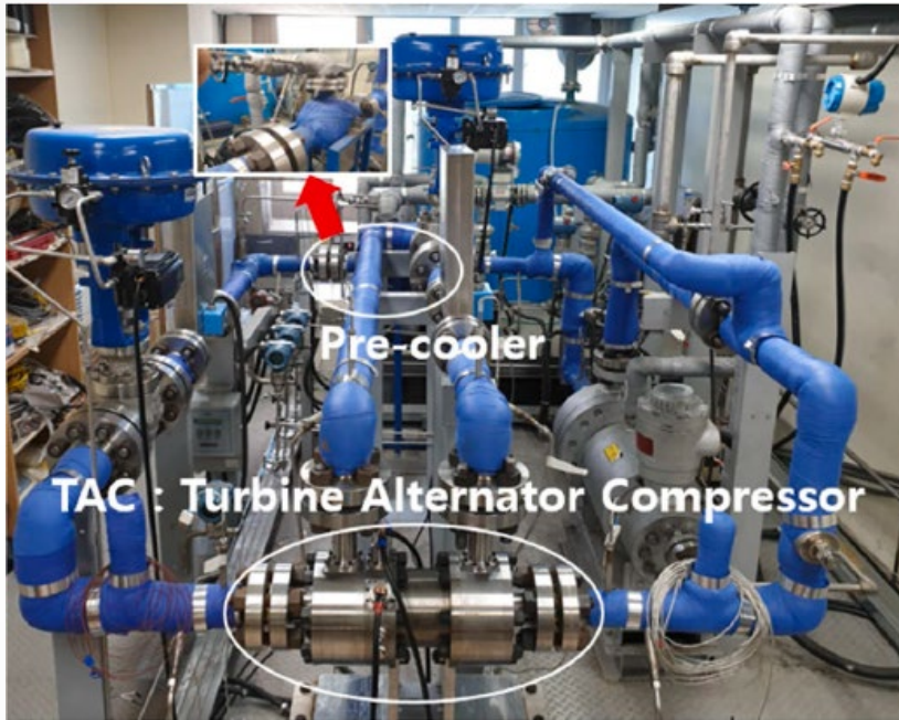
< S-CO 2 compressor test loop in KAIST >
