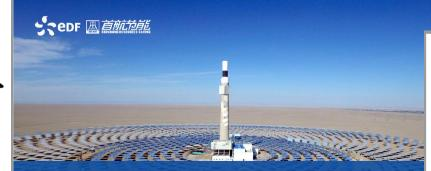
Retrofit of Dunhuang 10 MW molten salt plan with a high temperature supercritical CO<sub>2</sub> cycl
