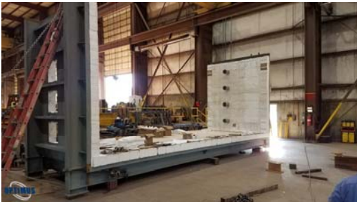
Burner Section module being fabricated
